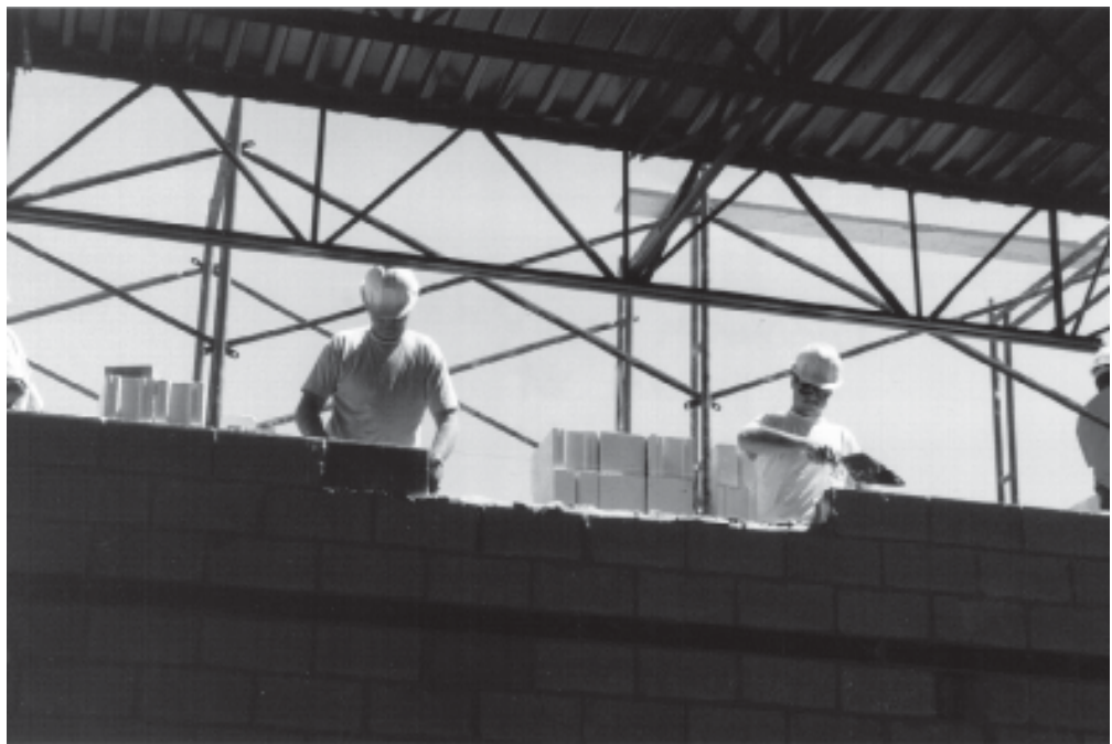
Placement of Concrete Masonry Units
