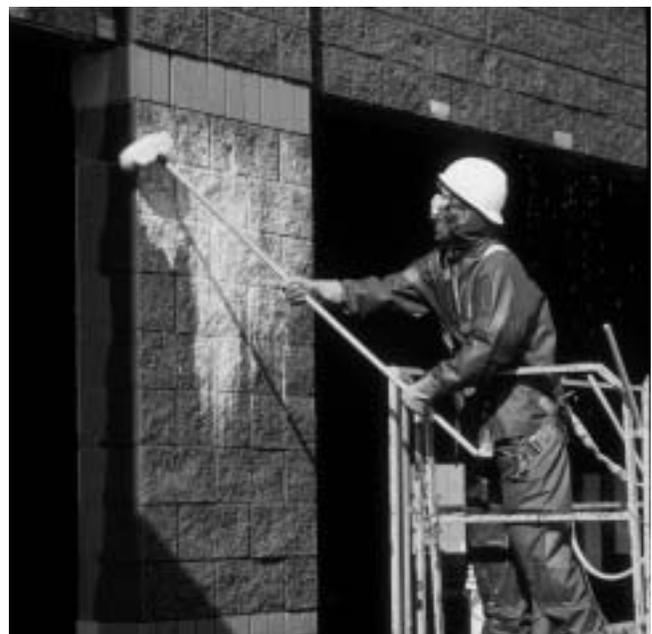
**Figure 1—Pressure Chemical Cleaning**
