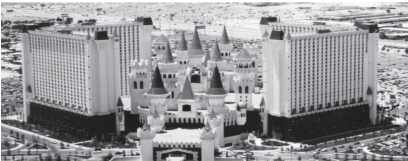
Figure 1—The four towers of the 28-story Excalibur Hotel in Las Vegas are load-bearing masonry.
