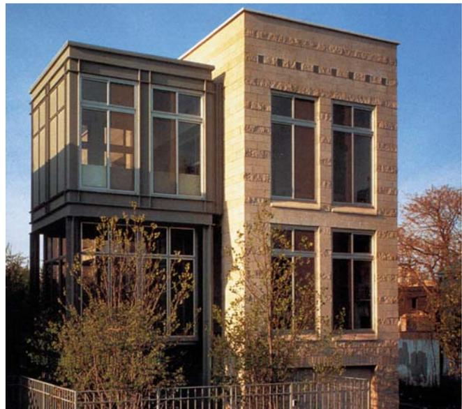
**Figure 1—Exterior Concrete Masonry in a Residence**
