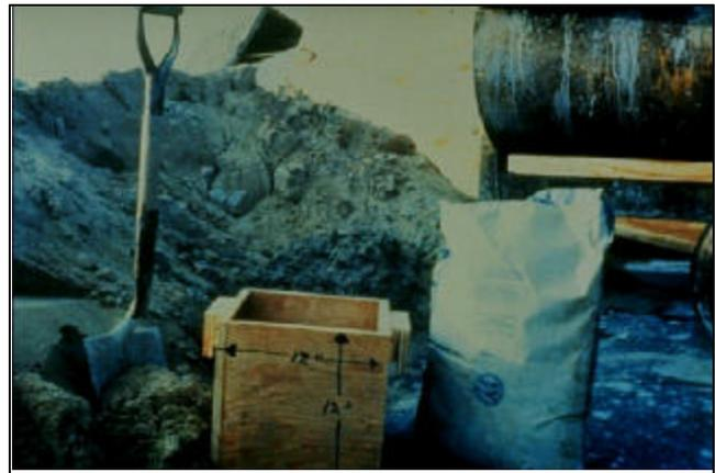
**Figure 1—Measuring Mortar Sand Volume**
